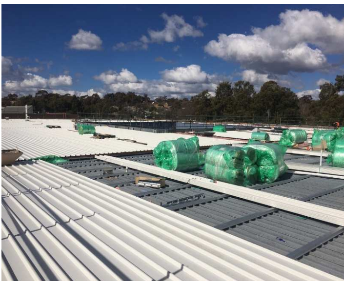
Progress photo of roof sheet and insulation installation.
