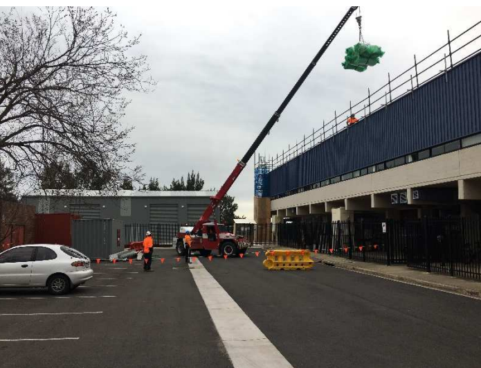
Progress photo of insulation being loaded to the roof for installation.
