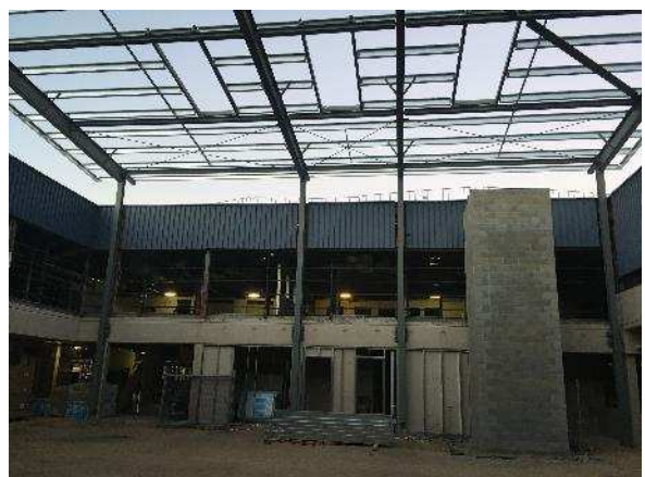
View of Stage 1 works from the internal courtyard.
