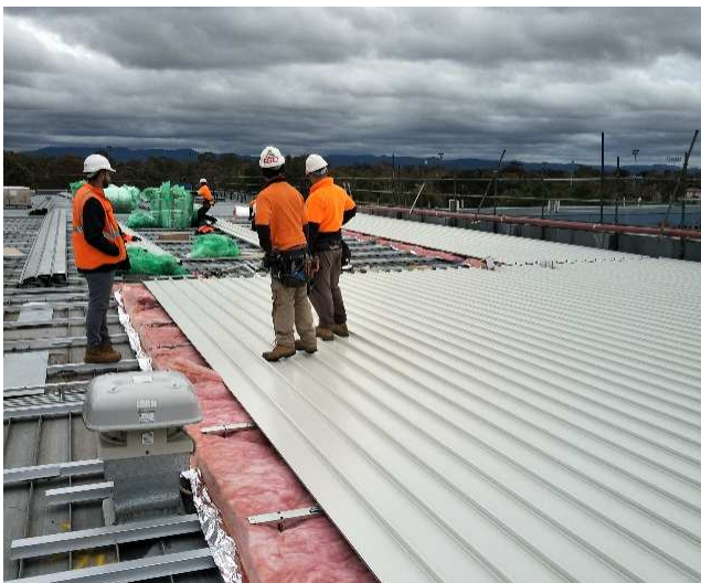
Progress photo of insulation and roof sheet installation.
