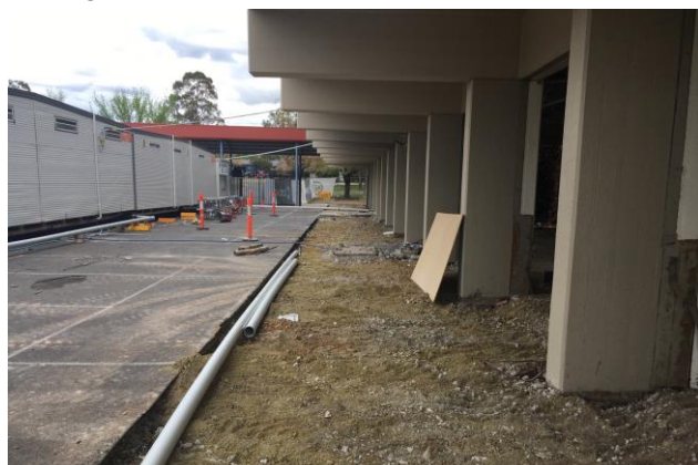
Demolition works continuing to the extent of the building line.
