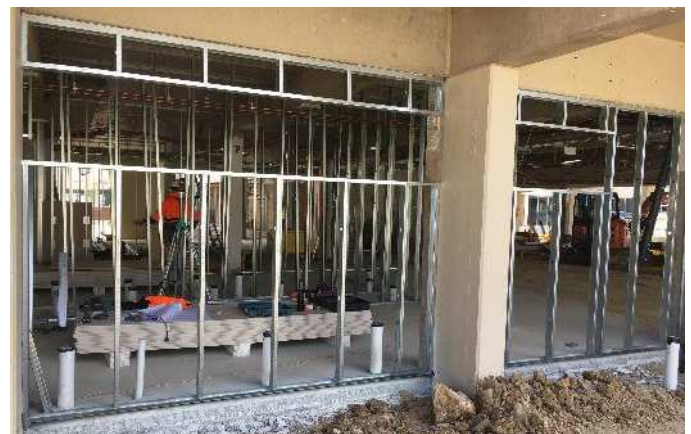
Framing install for ground floor external walls.
