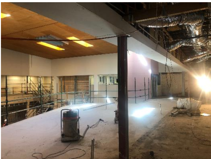
Curved overhang slab with lift installed
