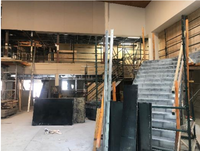
Stair 1 in the Learning Commons after pouring
