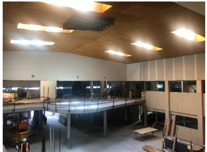
Internal courtyard works underway
