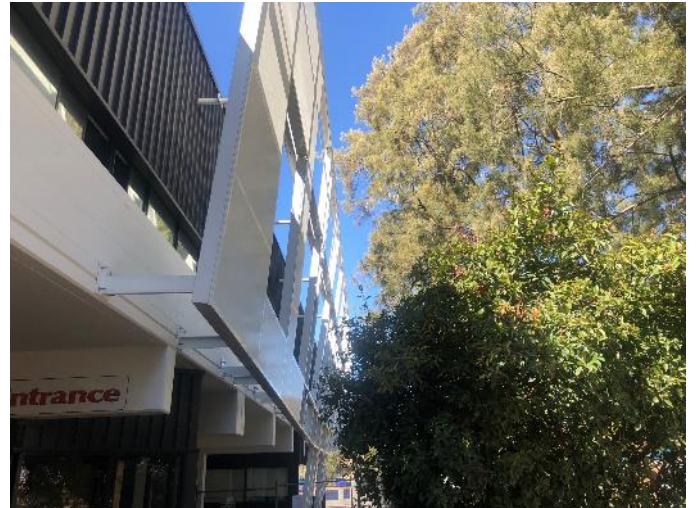
Structural steel works for façade screen underway
