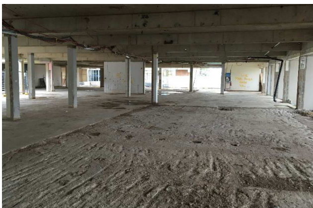
Ground floor demolition progress with structural elements in place..
