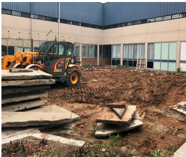
Current progress photo of completed courtyard works
