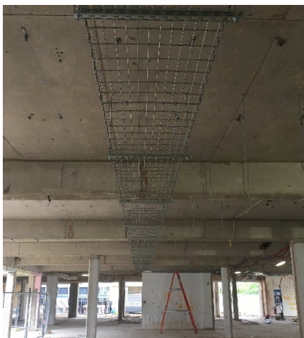
Demolition of concrete upstands on the courtyard side of Stage 1.
